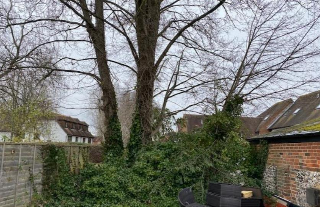
View of TPO group and curtilage listed boundary
