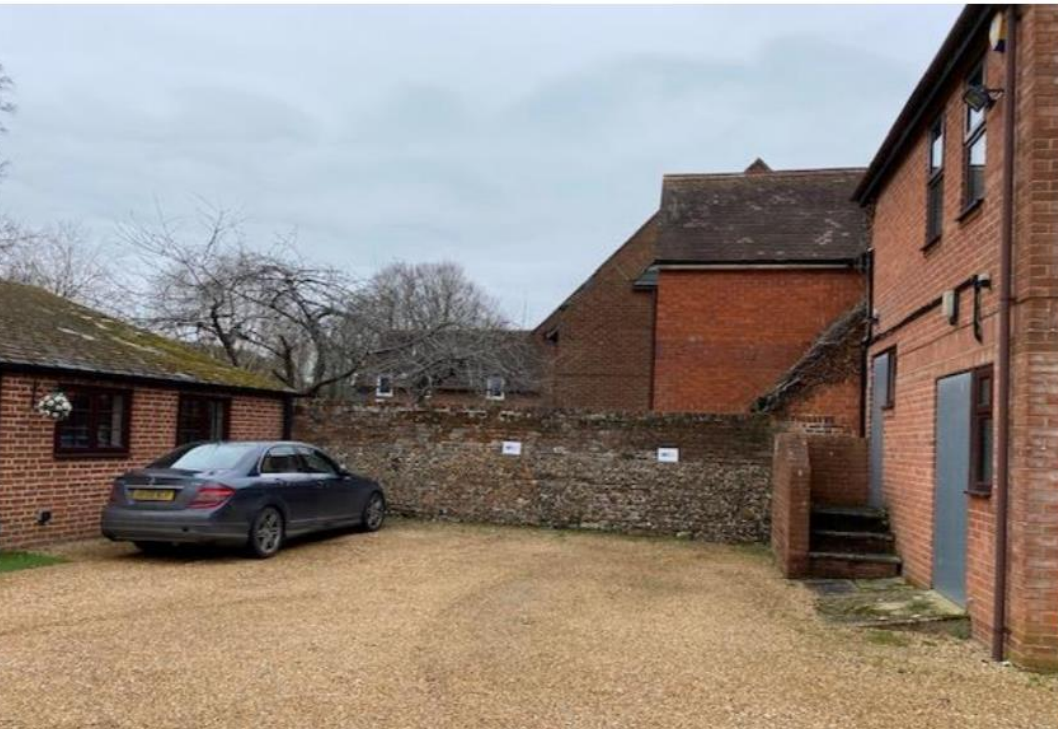
View of curtilage listed wall
